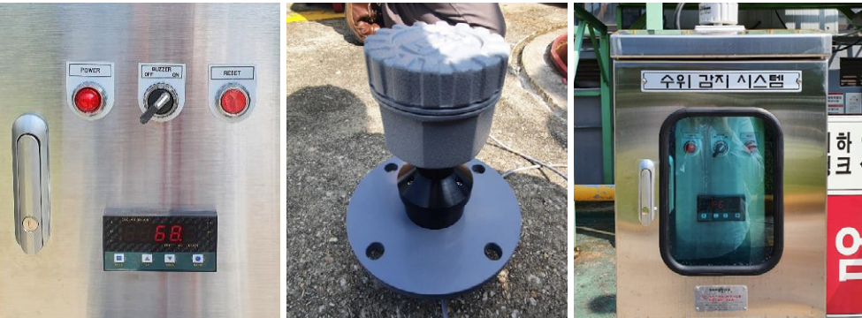
The ultrasonic liquid level gauge in the storage tank and the alarm for preventing overcharging
